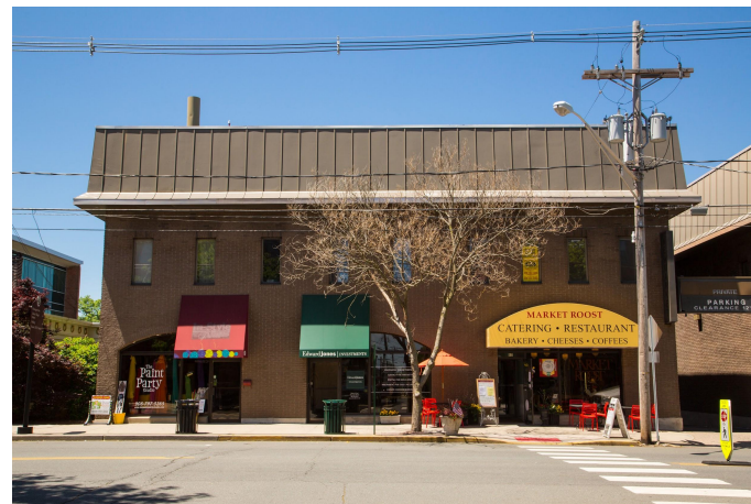
Location: Flemington, NJ Description: 6'-6" tall, 18" O.D.
